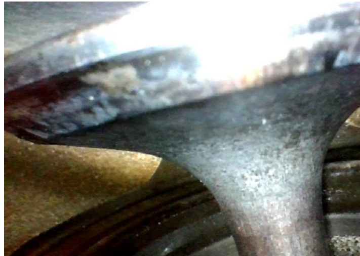
Photo above: Valve inspection
